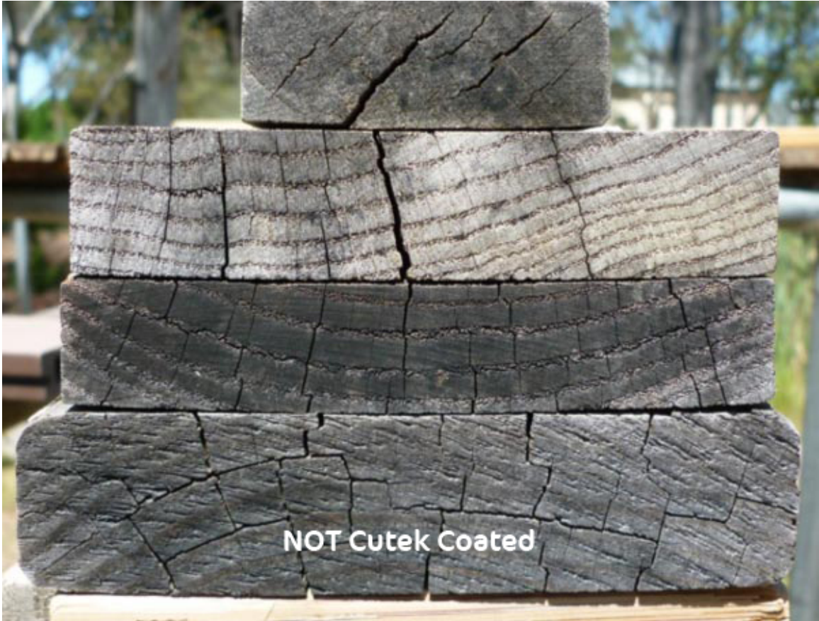
Picture 4 The same pieces of lumber as in Picture 3, showing the uncoated ends, after 12 months of full sun and rain exposure.
